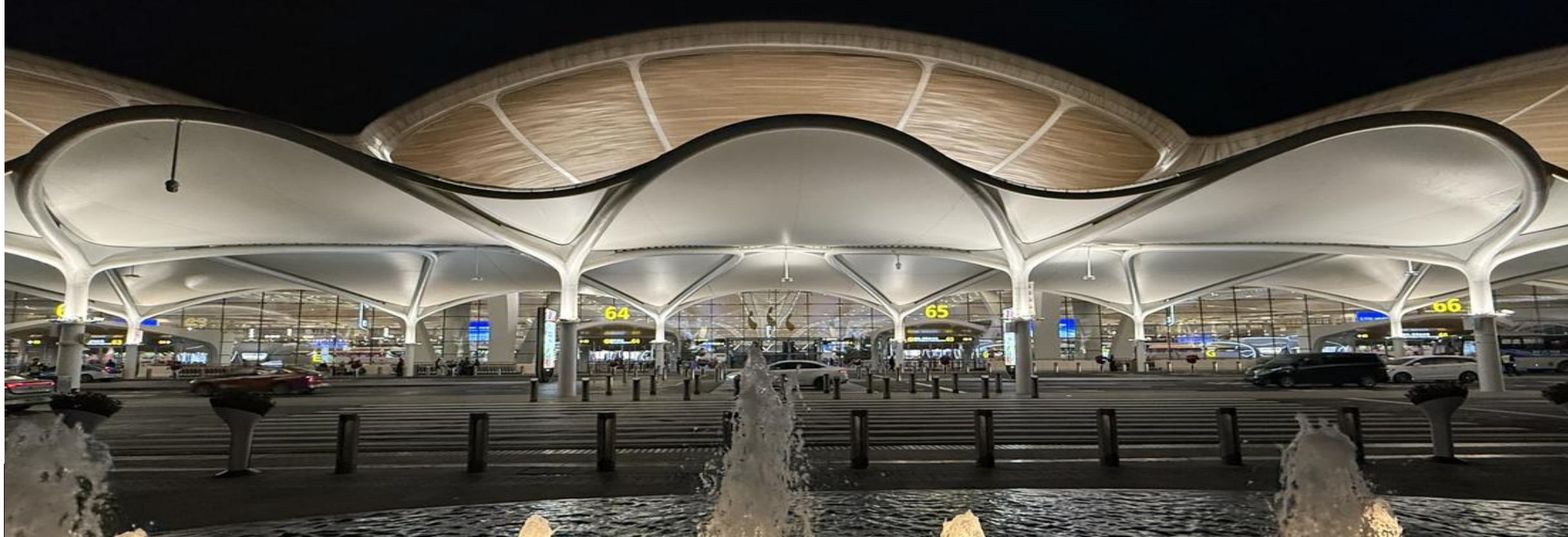
Guangzhou Baiyun Airport, Guangzhou. Chine
